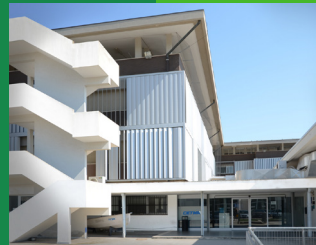
Site 5: CETMA & E@W Building Brindisi, Italy
